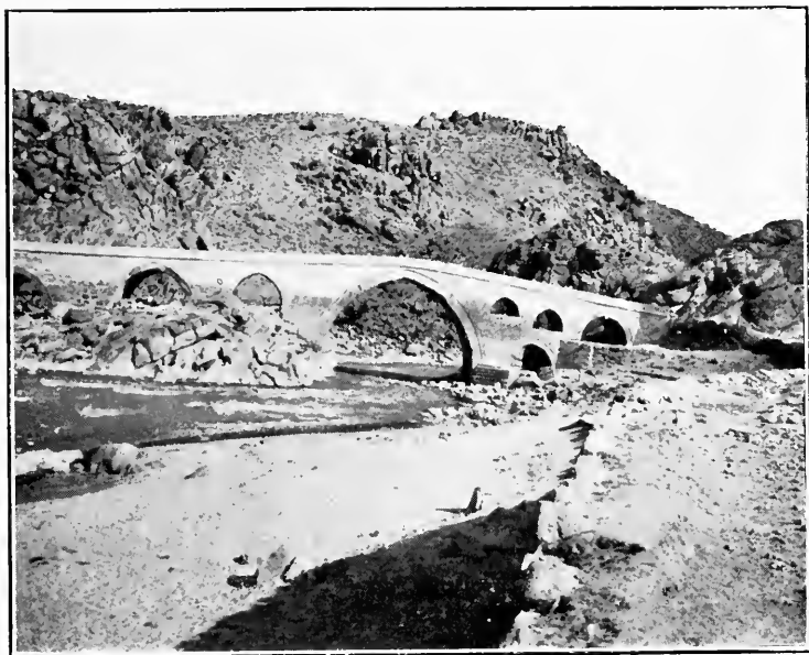
BRIDGE AT KEUPRI KEUI
